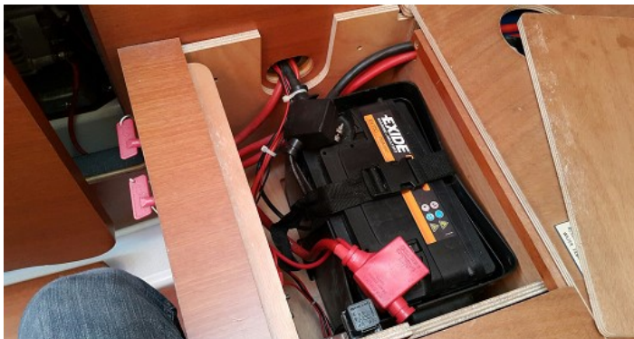
The servise and engine battaries main breaker with red key are located on the wall aft port cabin .
