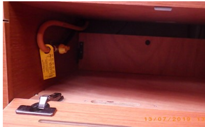
Gas valve under the stove
