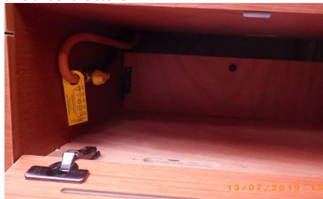
Gas valve under the stove
