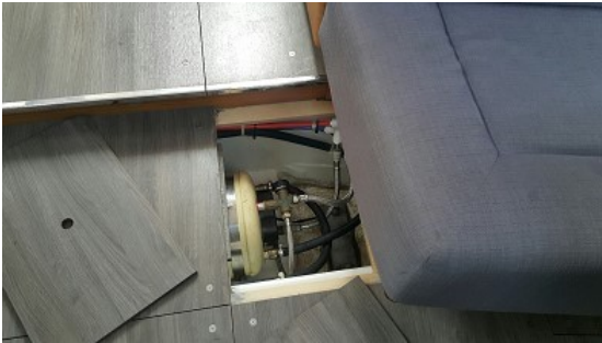
Water heating switch
