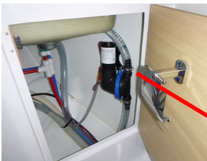
Shower pump switch
