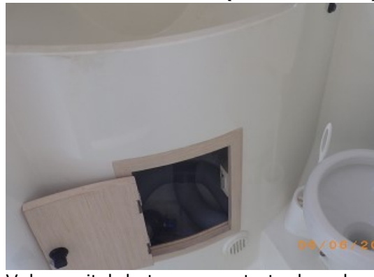
Starboard WC valve outlet (with waste tank)
